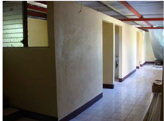
Urgent Care Unit under construction
